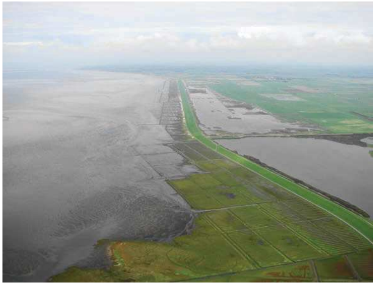
Figure 4.1: Dike built in 1980/81 at the Danish-German border of the Wadden Sea to shorten and strengthen the line of defence. The embanked area is maintained as a semi-natural wetland. In front of the dike, a foreland has been developed to dissipate wave energy. Further off the dike, natural saltmarsh succession has commenced (lower left), (Photo: K. Reise).
